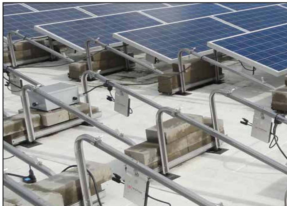
Microinverters Mounted to Racks Beneath Solar PV Panels
